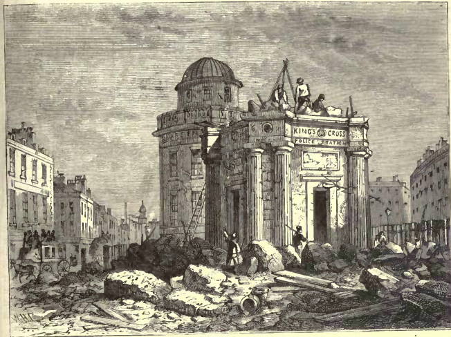
KING'S CROSS. From a View taken during its demolition in 1845. (See page 278.)
